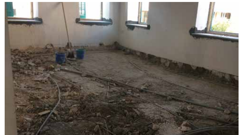
Figure 16a/b/c/d: Removal of damaged Cyprus marble flooring in the first-floor entrance hall and deteriorated non-original timber elements in Room 5 (Menteş, 2016)
