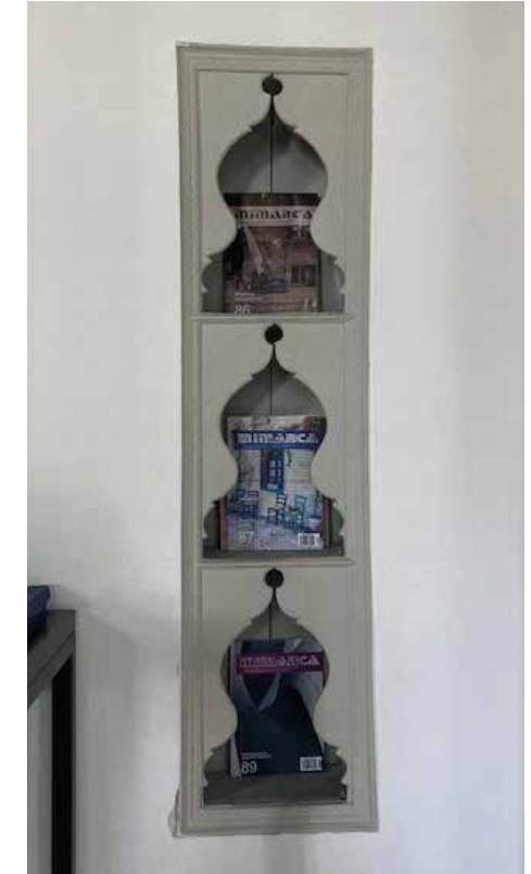
Figure 22: Wooden niche in the upper-floor room after restoration (Menteş, 2017)
