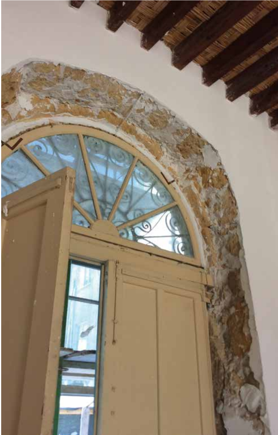
Figure 12g: The pre-restoration condition of the front door (Menteş, 2015)
