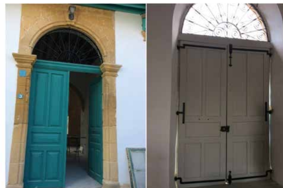
Figure 18a/b: Exterior and interior views of the entrance door before and after restoration (Menteş, 2017)
