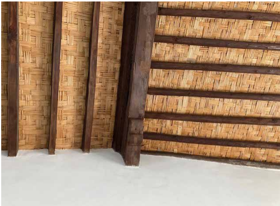
Figure 23a/b: Condition of timber ceiling, rafters, and woven cane after conservation (Menteş, 2017)
