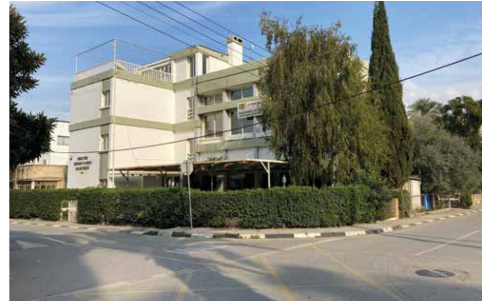
Figure 2: The first premises of the Building of UCCTEA Union Building, located in the Çağlayan Neighbourhood, Şehit İbrahim Ali Street, Nicosia (Menteş, 2020)
