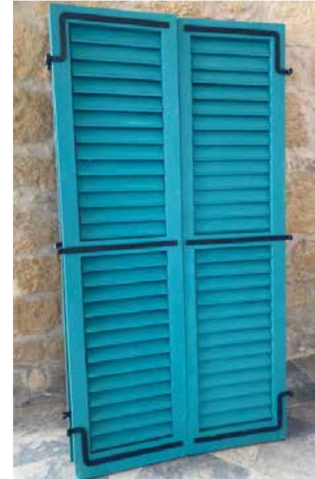
Figure 21: Shutters after restoration, before installation (Menteş, 2017)
